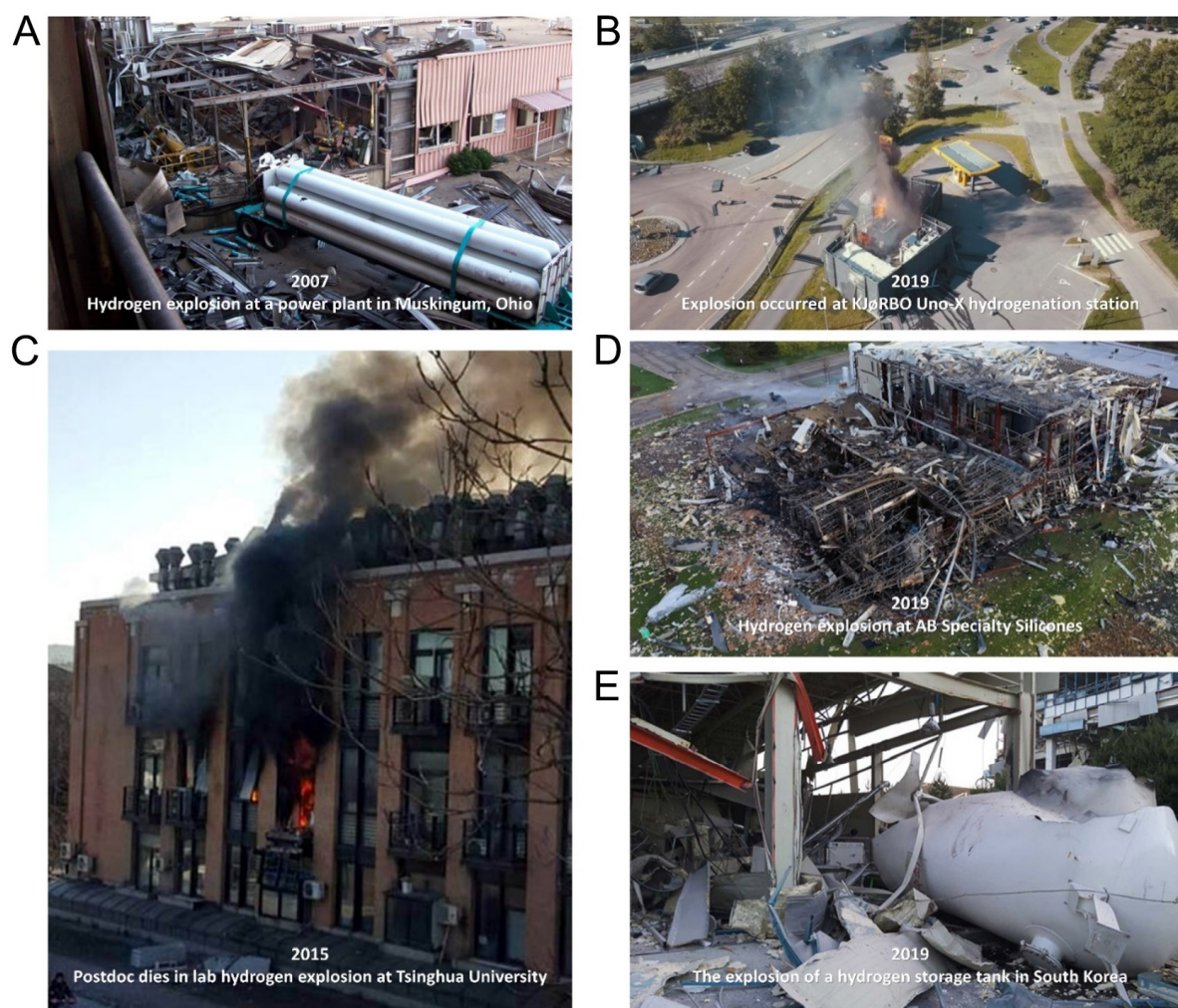
Figure 1. Typical hydrogen incidents. (A) A fatal hydrogen explosion at a power plant in Muskingum, Ohio. (B) A hydrogen explosion occurred at KJØRBO Uno-X hydrogenation station in Sandvika, Norway. (C) Laboratory hydrogen explosion in Tsinghua University. (D) An explosion at AB Specialty Silicones in Waukegan, Illinois. (E) Damage to nearby buildings after the explosion of a hydrogen storage tank in South Korea.
