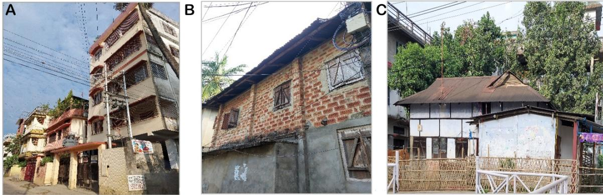
**Figure 2.** Observed MBTs (A) RC, (B) unreinforced masonry, and (C) Assam-type buildings at Silchar City.
