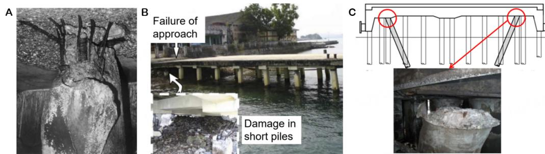
**Figure 1.** Seismic damage to wharf pile foundations. (A) 1989 Loma Prieta earthquake<sup>[3]</sup>; (B) 2004 Sumatra earthquake<sup>[4]</sup>; (C) 2010 Maule earthquake<sup>[7]</sup>.
