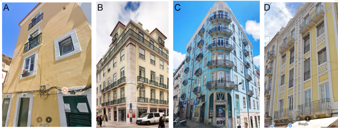
Figure 1. Typology of Portugal's historic masonry buildings: Pre-Pombalino, Pombalino, Gaioleiro, and Placa. It highlights the characteristics and structural features of each typology, emphasizing their historical significance and variations in construction methods.
