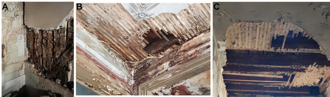
Figure 6. Severe situations and deteriorated parts: Interior wall (A), roof (B), and floor (C).
